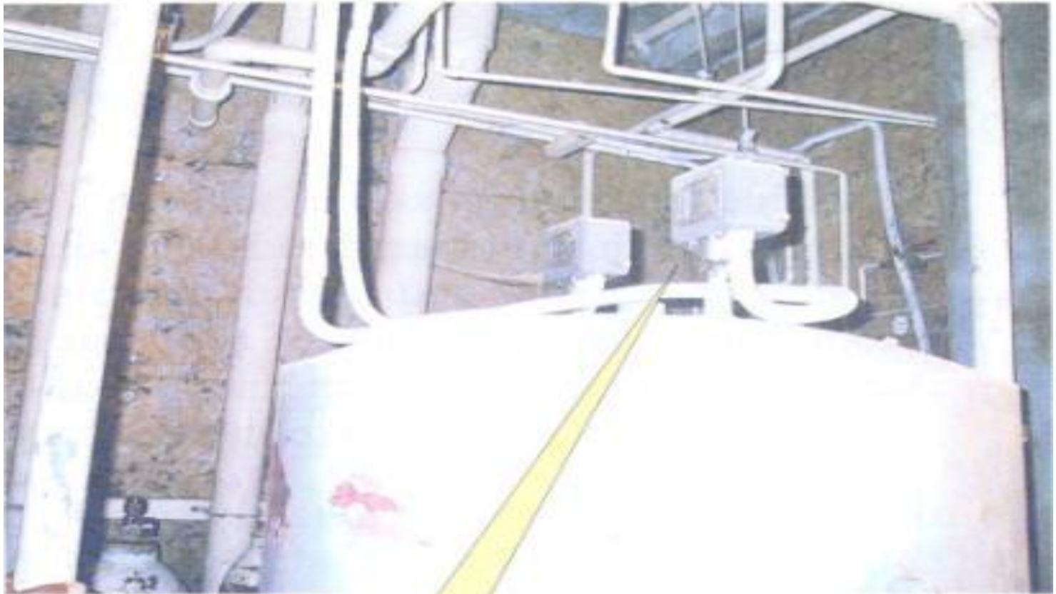
Flexible pipe connected with heavy equipment
